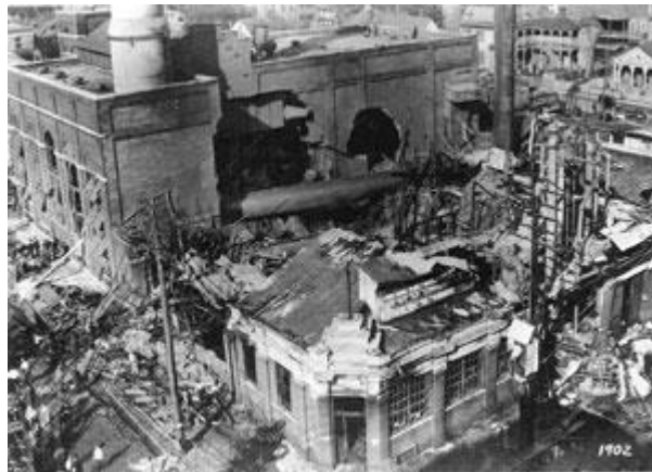
Figure 2. Effects of a Boiler Explosion
