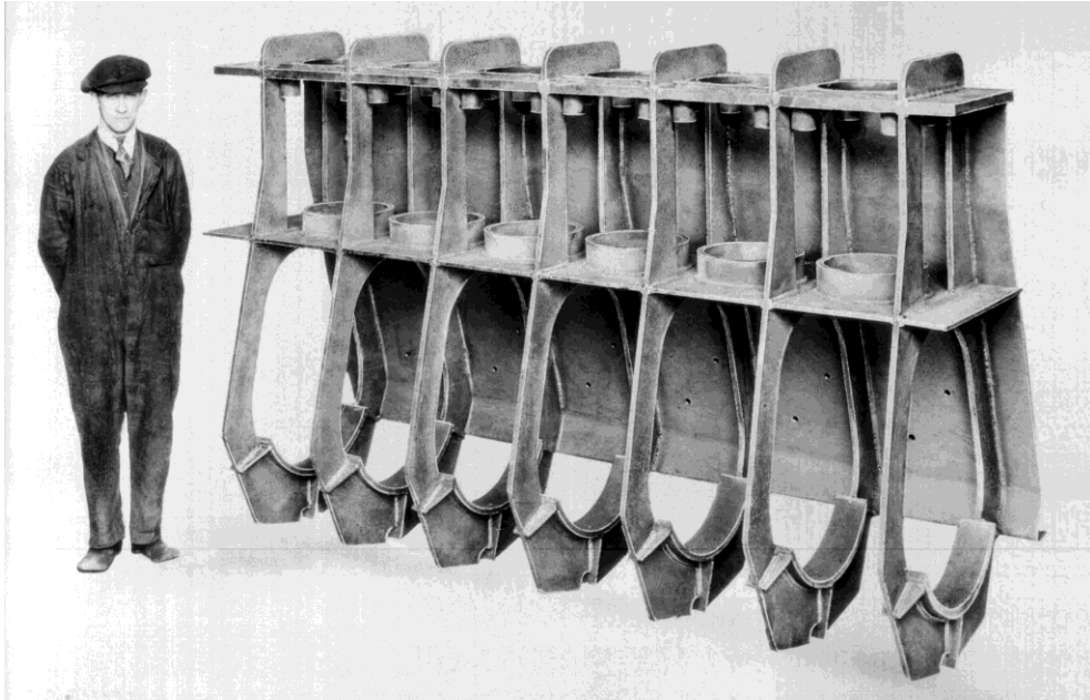
Figure 6. Stevens' patent welded steel engine frame.
